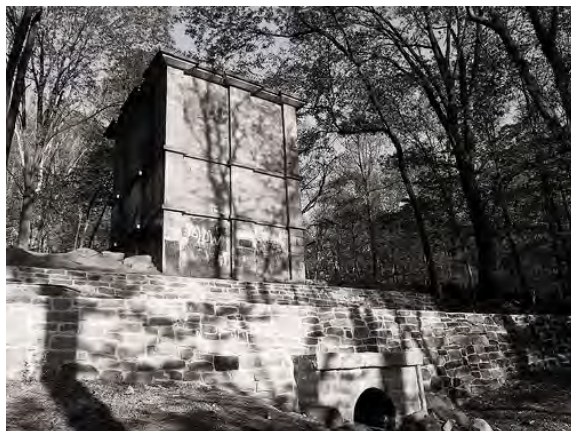
Old weir at the Croton Aqueduct, Source: http://imjustwalkin.com/
