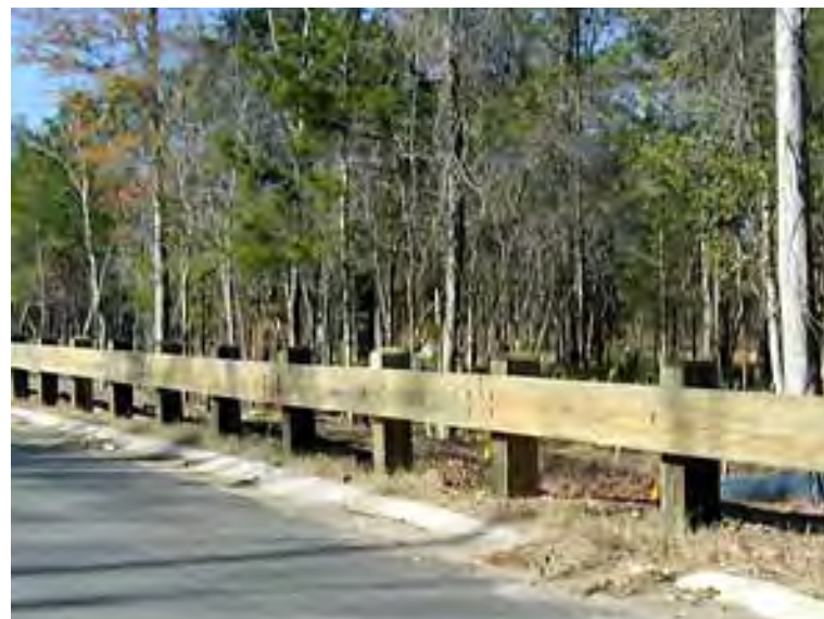
Timber guardrails along paved roads around the park.
