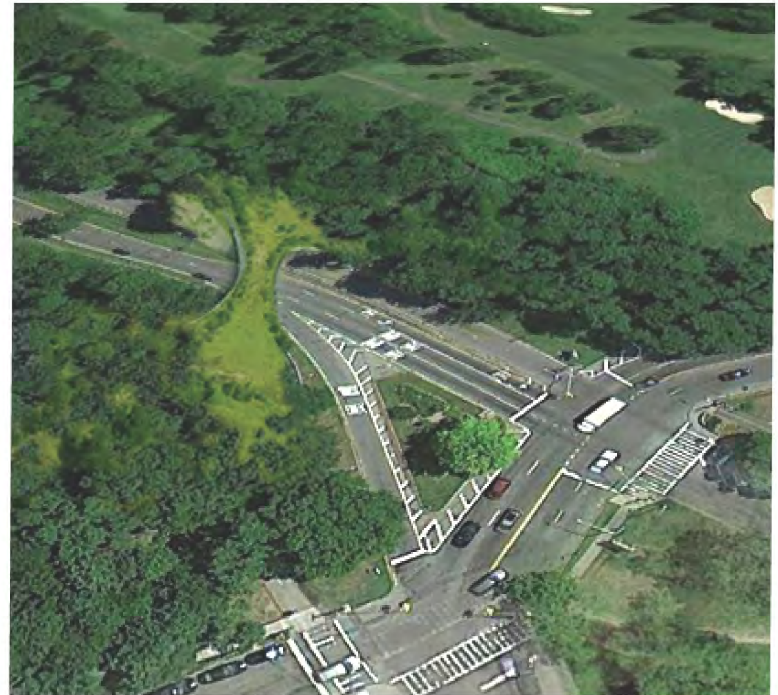
Proposed landbridge enabling pedestrians, golf carts, and wildlife to cross over Mosholu Parkway.
