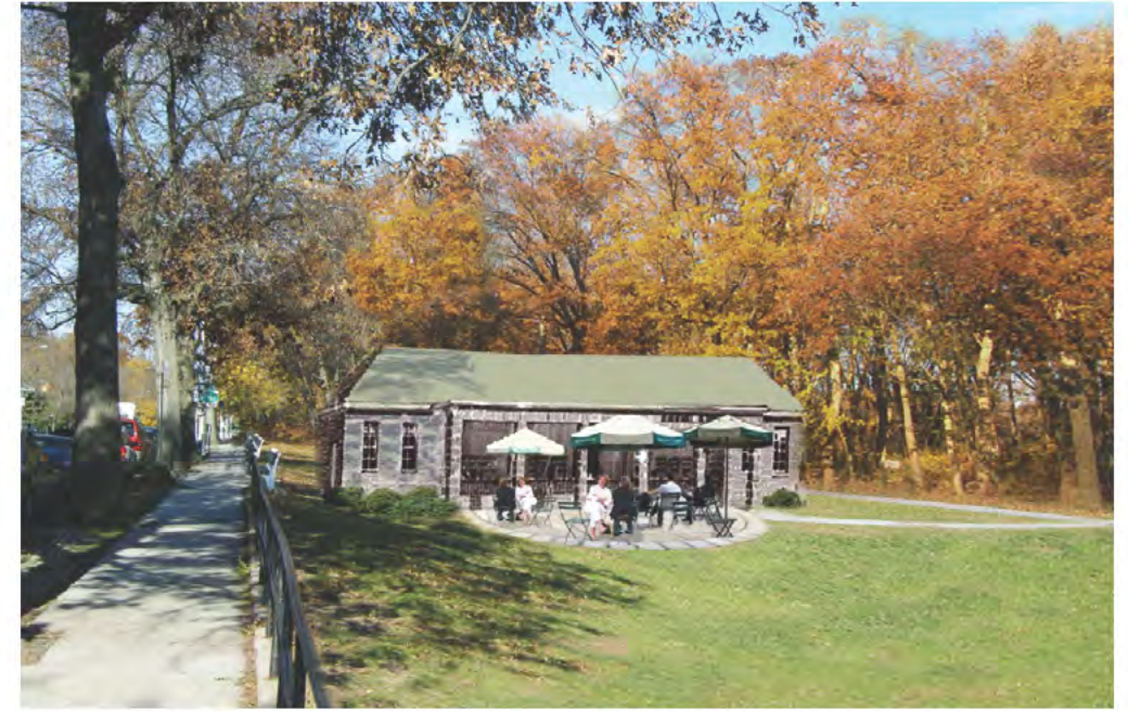
Proposed comfort station and food concession at the north edge of the Parade Ground.
