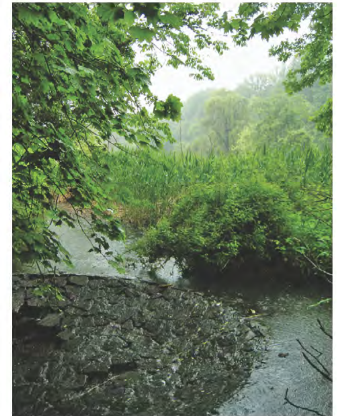
Tibbetts Brook showing siltation caused by culverts .
