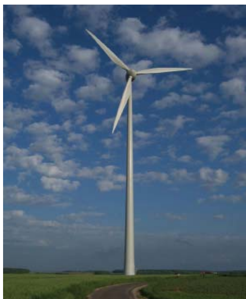
Four or five large turbines, like this one, may be able to generate enough energy to provide power to the entire park.
