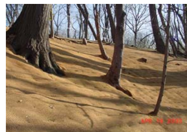
3) Slope stabilization at Riverdale Park
