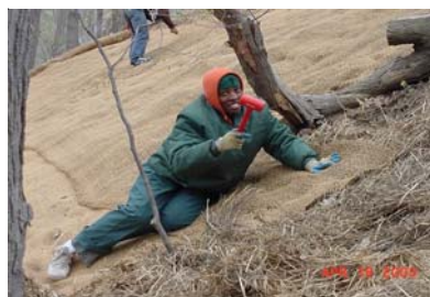
17) POP participant installing erosion fabric
