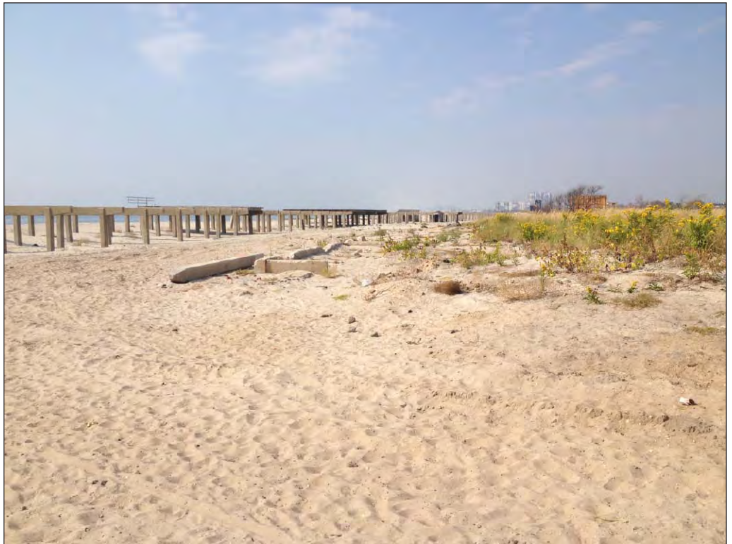
View of the maritime beach and maritime dunes communities, and boardwalk foundation near Beach 36th Street, facing west
