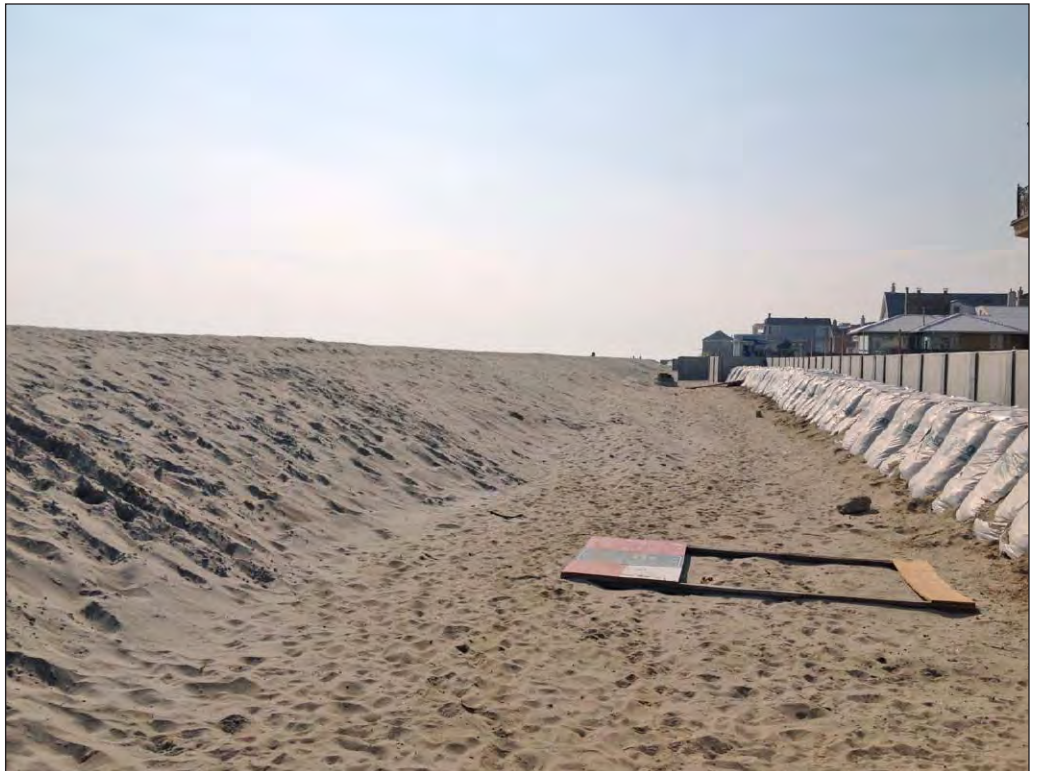
View of the USACE berm to the left near Beach 145th Street, facing west
