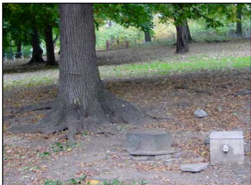
Eroded soils on the eastern hillside expose once buried tree roots and concrete drain box and deposit silt on the stairs and sidewalk.
