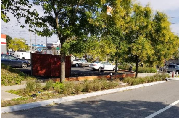
Top: Stormwater Greenstreet built at the intersection of Van Duzer Street and Targee Street.
