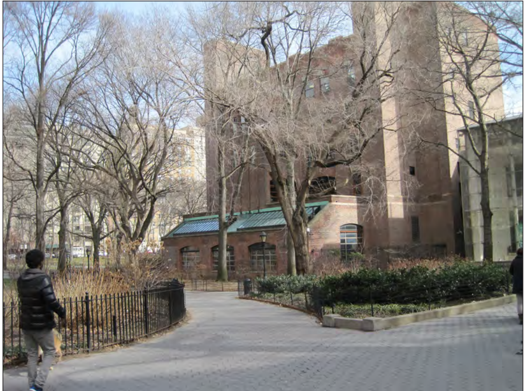
AMNH. Former power house. View northeast 3
