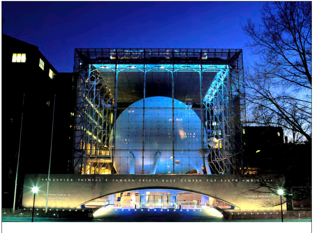
Evening View of Rose Center Entrance
