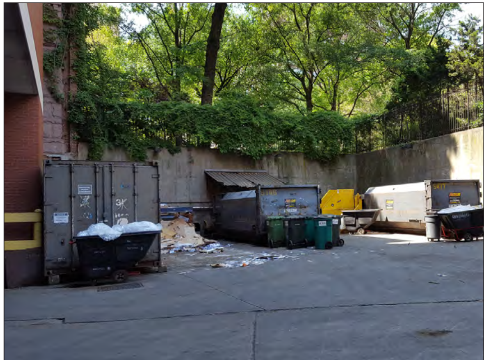
View west towards the Museum's refuse/dumpster area located in the service yard of the Museum 12
