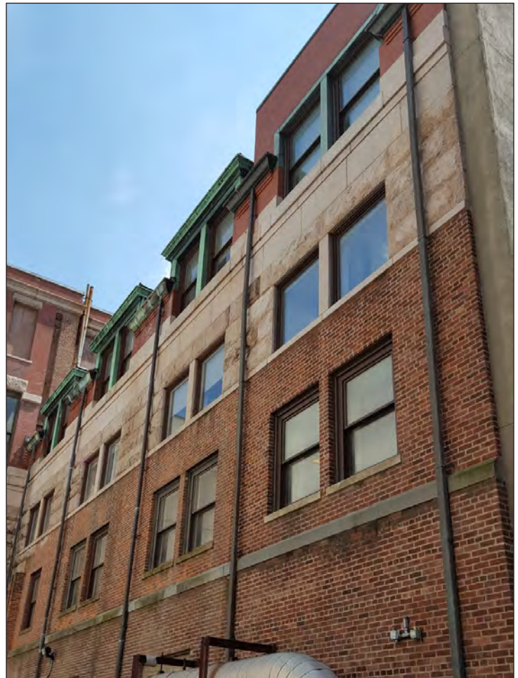
View of the north façade of Building 15 10
