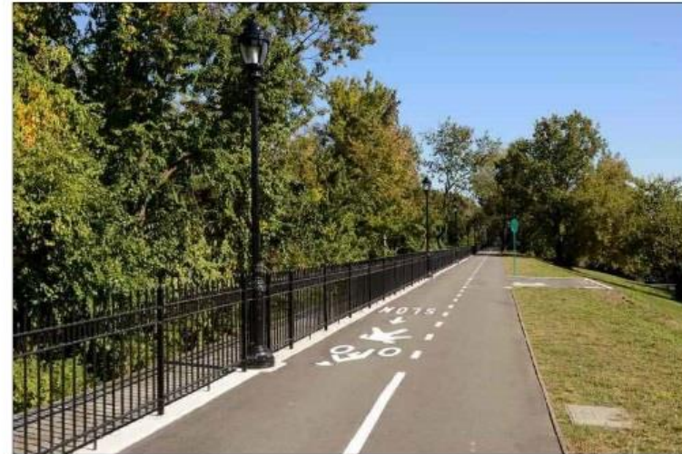
4. INSTALL 4' FENCE WITH PICKETS.
