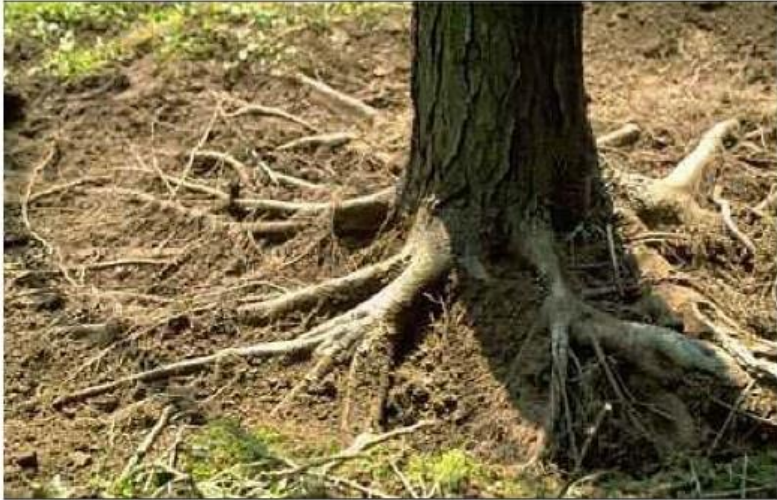
1. REMOVE SOIL BY HAND AND VACUUM IN PLANTING STRIPS (0-6").
