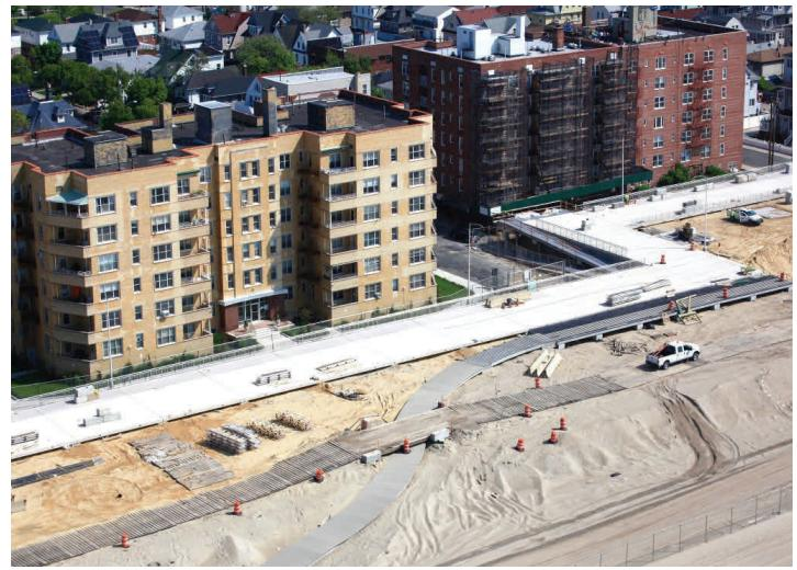
Phase 3A— Precast Plank Grouting & Railings
