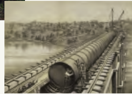
Laying large pipe across the High Bridge, 1861-62
