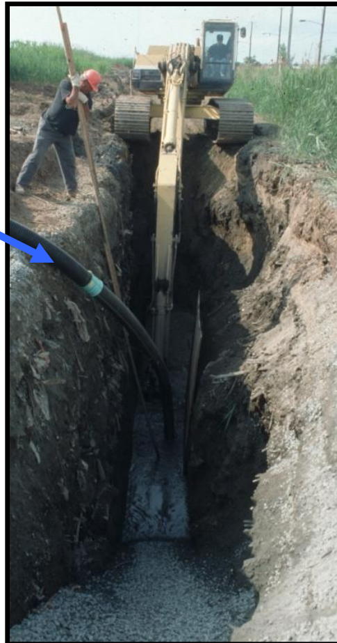
Leachate Collection Drain Construction
