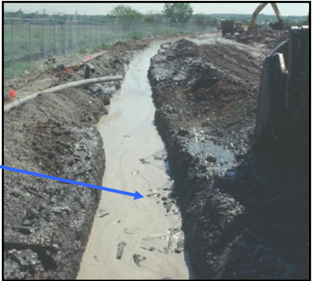
Typical Cutoff Wall Construction
