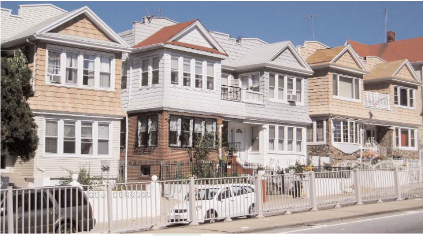
Attached houses line a hillside as the Greenway heads to Highland Park.
