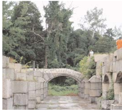
The fortifications of Fort Totten, now New York City parkland
