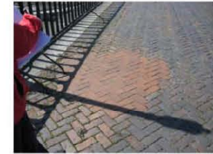
Example of non-matching brick patch circa 1970s
