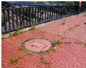
Manhole cover installed at vault light opening in metal span
