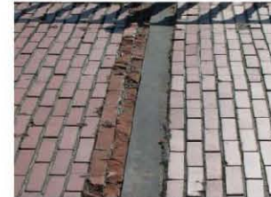
Expansion joint detail at steel span center hinge
