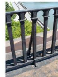
Out-board bracing at 1928 rail
