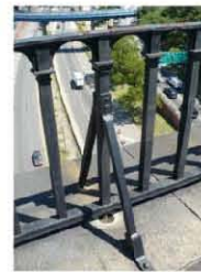
In-board (non-original) and out-board rail bracing at 1850 rail
