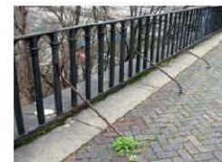
Non-original in-board bracing at 1864 rail
