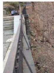
Typical Brace at 1850 rail, set in granite coping
