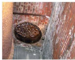
Cast iron vault light seen from bridge attic
