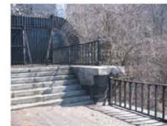
Missing cast iron scrolls at masonry abutment steps
