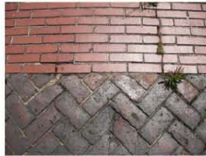
Juncture of 1862 herringbone paving & 1928 running bond paving
