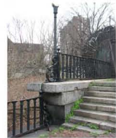
Cast iron light pole (1935 ca.) and cast iron scrolls at bridge steps
