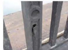
Cracked cast iron rail post at metal span
