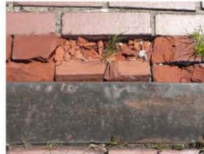
Deteriorated running bond brick units at expansion joint
