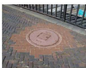
Manhole cover installed at vault light opening in masonry span
