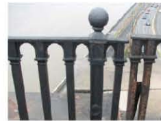
Non Historic cast iron finial (1979 ca.) at expansion joint
