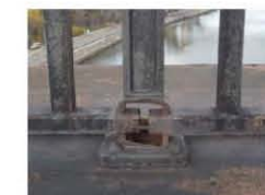
Deteriorated rail post base at metal span
