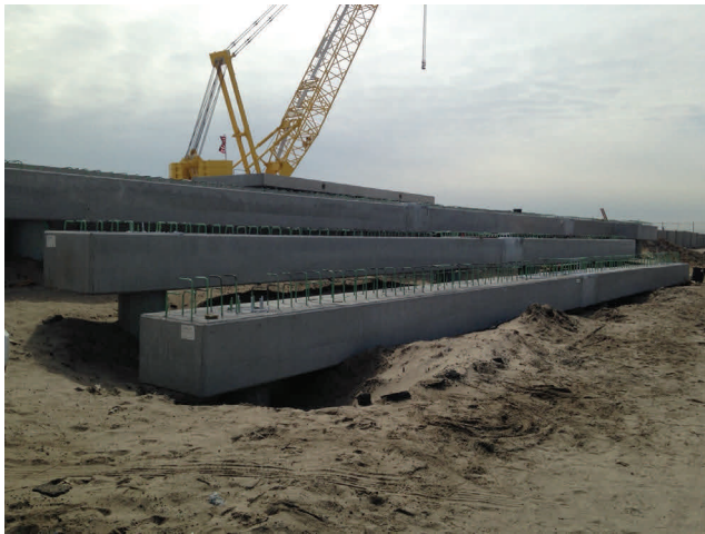
Phase 1 — Access Structure Pile Caps Installed
