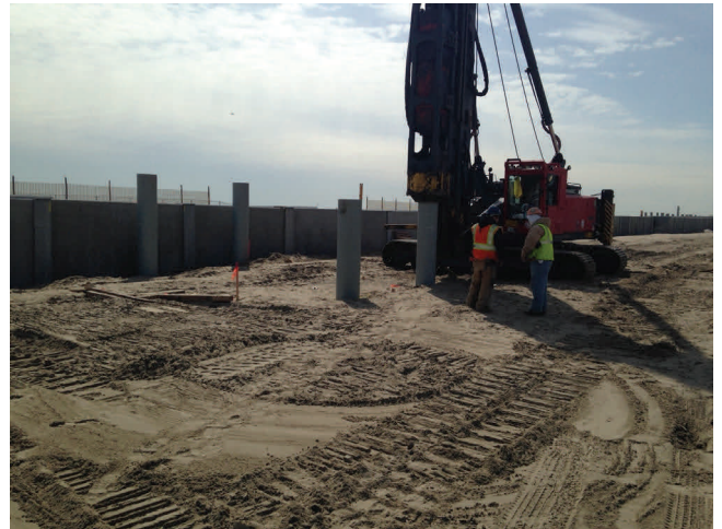
Phase 2— Access Structure Pile Driving
