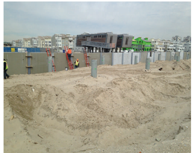
Phase 4B — Sand Retaining Wall Installation
