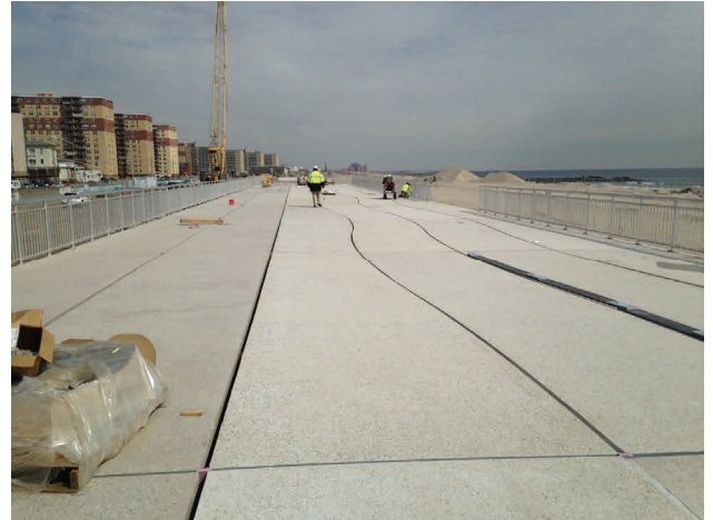
Phase 1— Precast Plank & Railing Install
