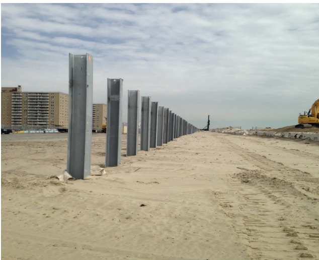
Phase 4A— Ongoing H Pile Driving
