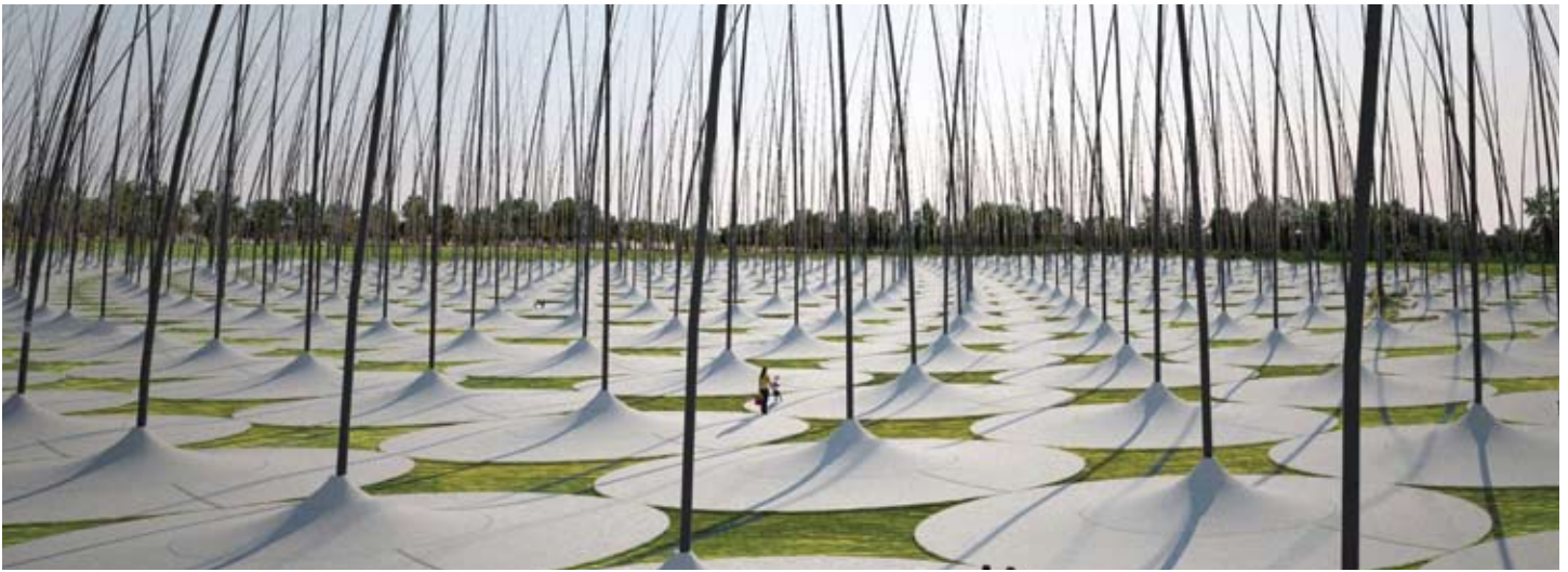
Above: A rendering of 'Windstalk', a 2010 LAGI competition entry that proposed a field of 55-foot tall carbon fiber stalks generating energy from the wind via piezoelectric and torque generators. Image courtesy of Society for Cultural Exchange
