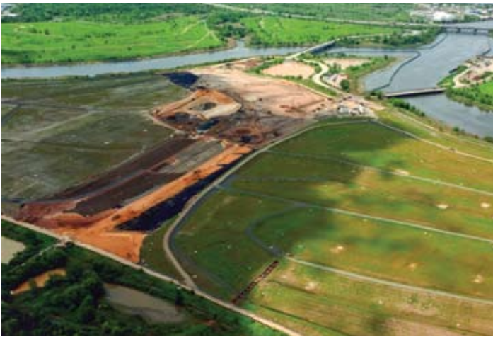
Left: DSNY's integration of sub-base for the Yukon Avenue road connection within the East Mound landfill cap saved the City millions of dollars in future work but required a host of changes to established capping procedures. Photo courtesy of Tully Construction. Right: A downchute on the East Mound allows large volumes of storm water run-off to rush down the slope toward detention basins during storms, without compromising the integrity of the landfill cap. Iron, washed out from the mound's soils and oxidized when exposed to air, has left the orange trail seen here. Official photo of NYC Department of Sanitation
